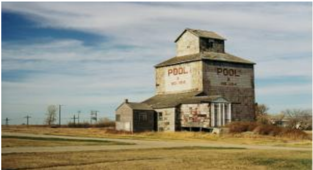
Built in 1895, this grain elevator in Fleming, Saskatchewan is the oldest existing elevator in western Canada
